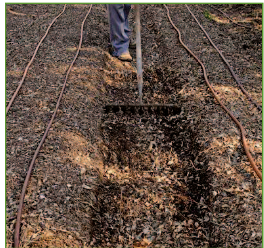
Figure 6. Cover the composting material with the original soil from the hole or trench.
